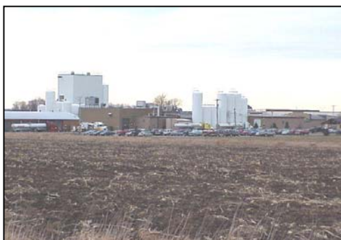
Grassland Dairy Butter Plant-Town of Eaton
